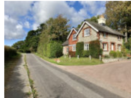
Entrance lodge to Purbrook Heath House
